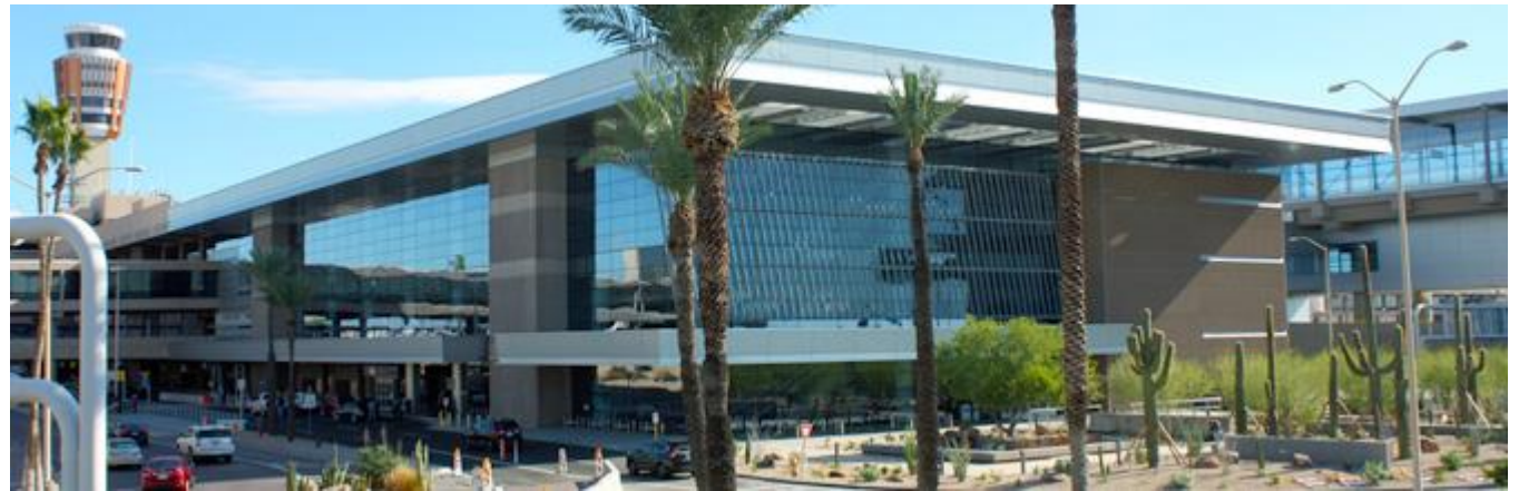
Photo of Terminal Modernization by Phoenix Sky Harbor International Airport. Retrieved from http://www.skyharbor.com/TerminalModernization
